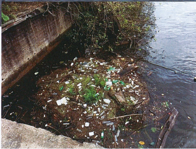
Photograph No. 9 – View of floating wood debris
